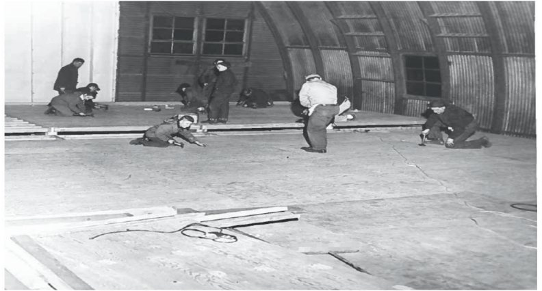
Construction on the quonset hut floor.
